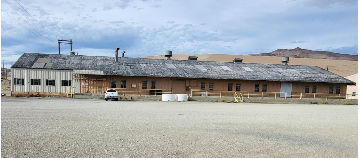
Figure 12-4: Yerington Copper Project Site Office, Core Logging, Sampling and Storage Facilities
